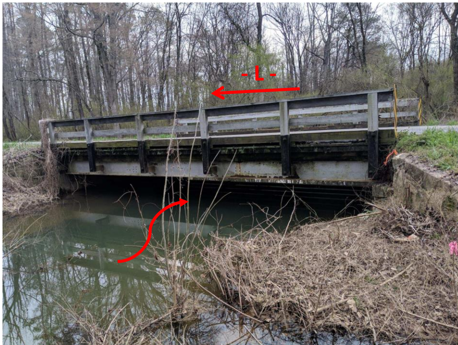
Photograph No. 2: View facing downstream.
